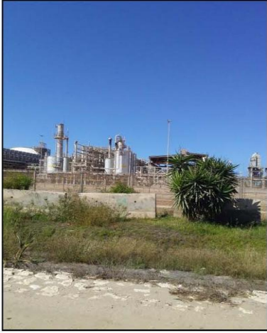
Photo.1. processing gas unit in idku plant Source: field study, 17 Oct. 2020.
